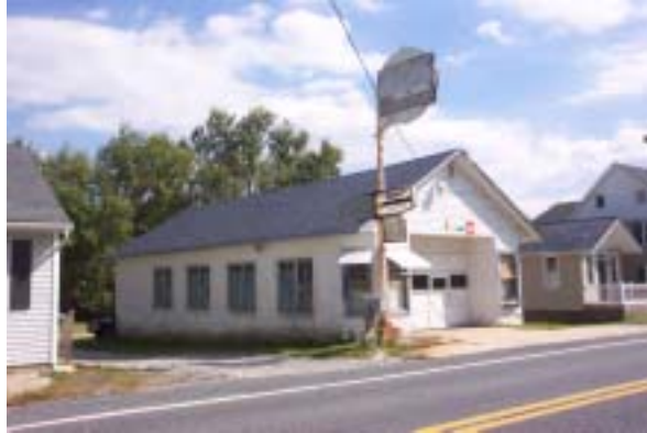
Picture 22: Norrisville's Freestanding Business Sign
