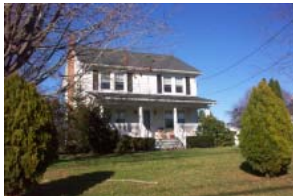
Picture 18: Front Porch Creates Semi Public Area on Front of Village Residence
