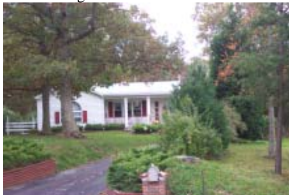
Picture 13: One Story Village Residence
