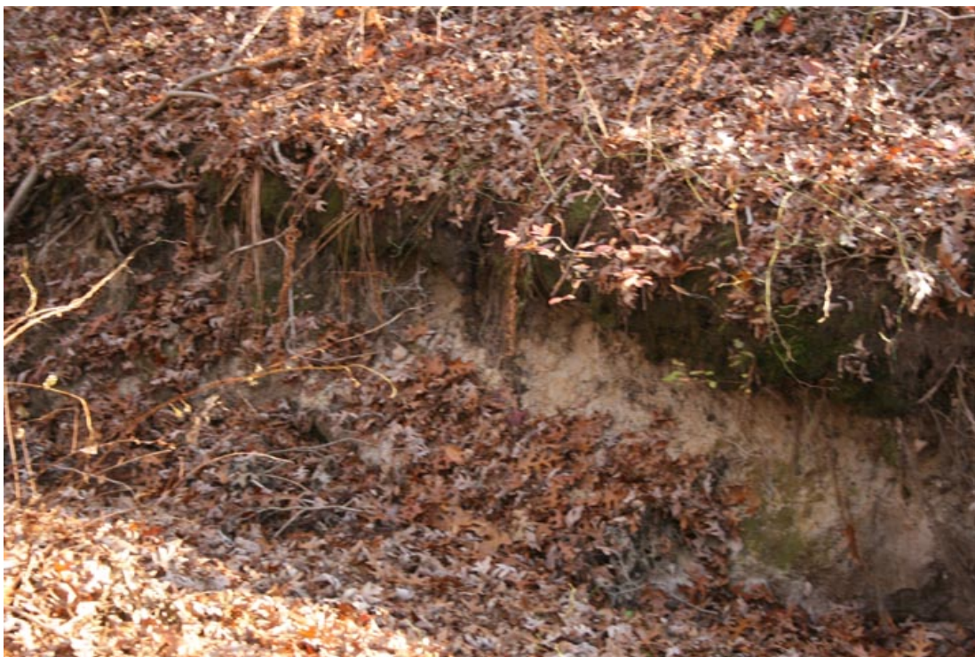
Photo 3.59 – Bank erosion along middle section of South Tributary
