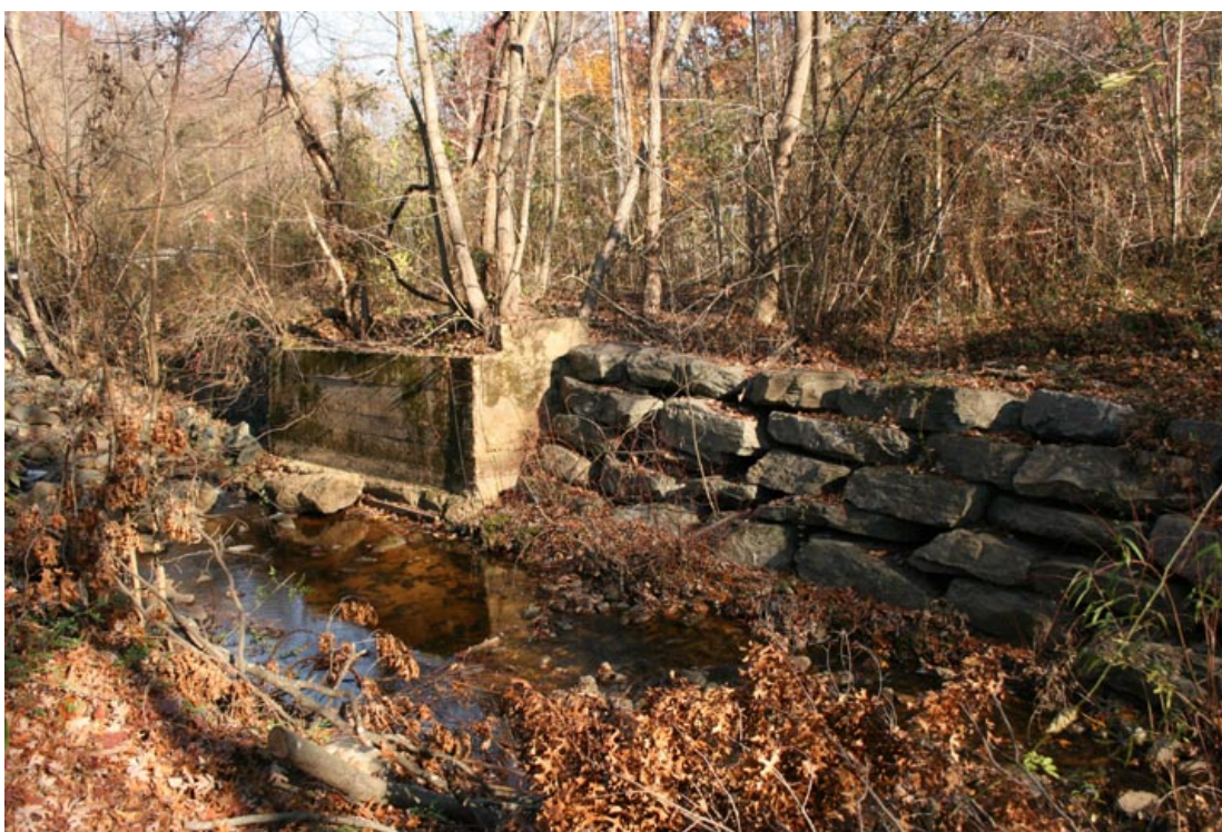
Photo 3.73 – Armoring along left bank of West Branch downstream of Trimble Road
