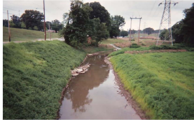
(b) Same reach four months after restoration with toe benches and soil fabric lifts. Note channel has been shifted away from failing slope and narrowed.
