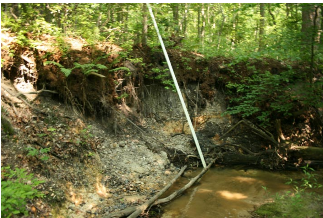
Photo 3.22 – Bank erosion along West Tributary
