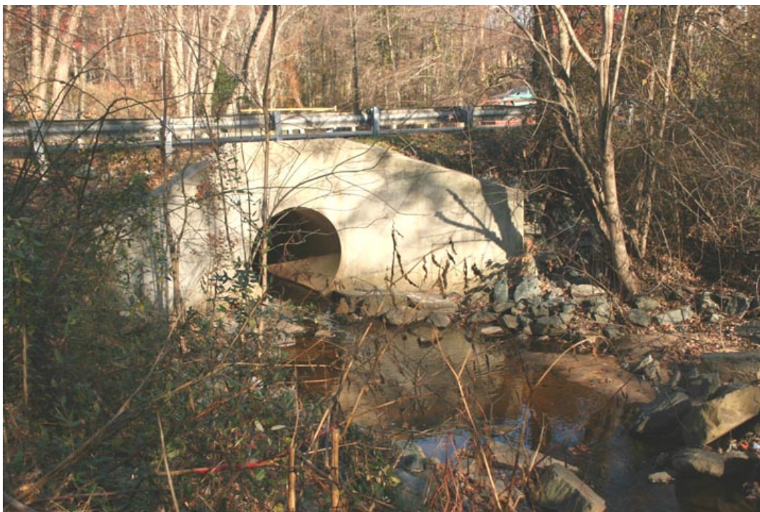
Photo 3.72 – West Branch culvert downstream side of Trimble Road
