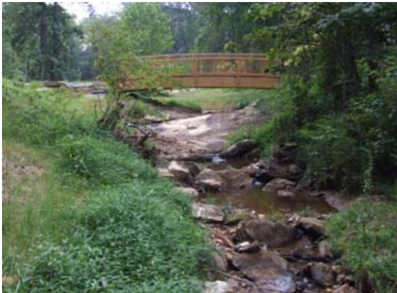
(b) Same reaches six months after restoration with log/boulder step-pools
