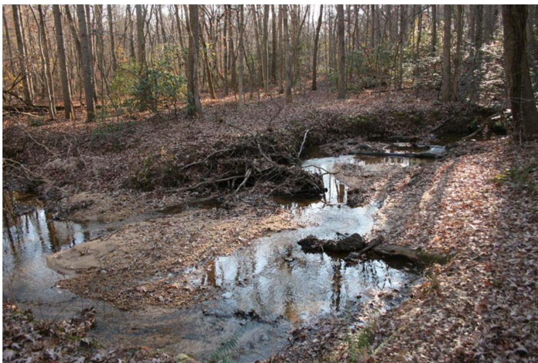
Photo 3.48 – Bank erosion, debris jams and bar deposition along upper section
