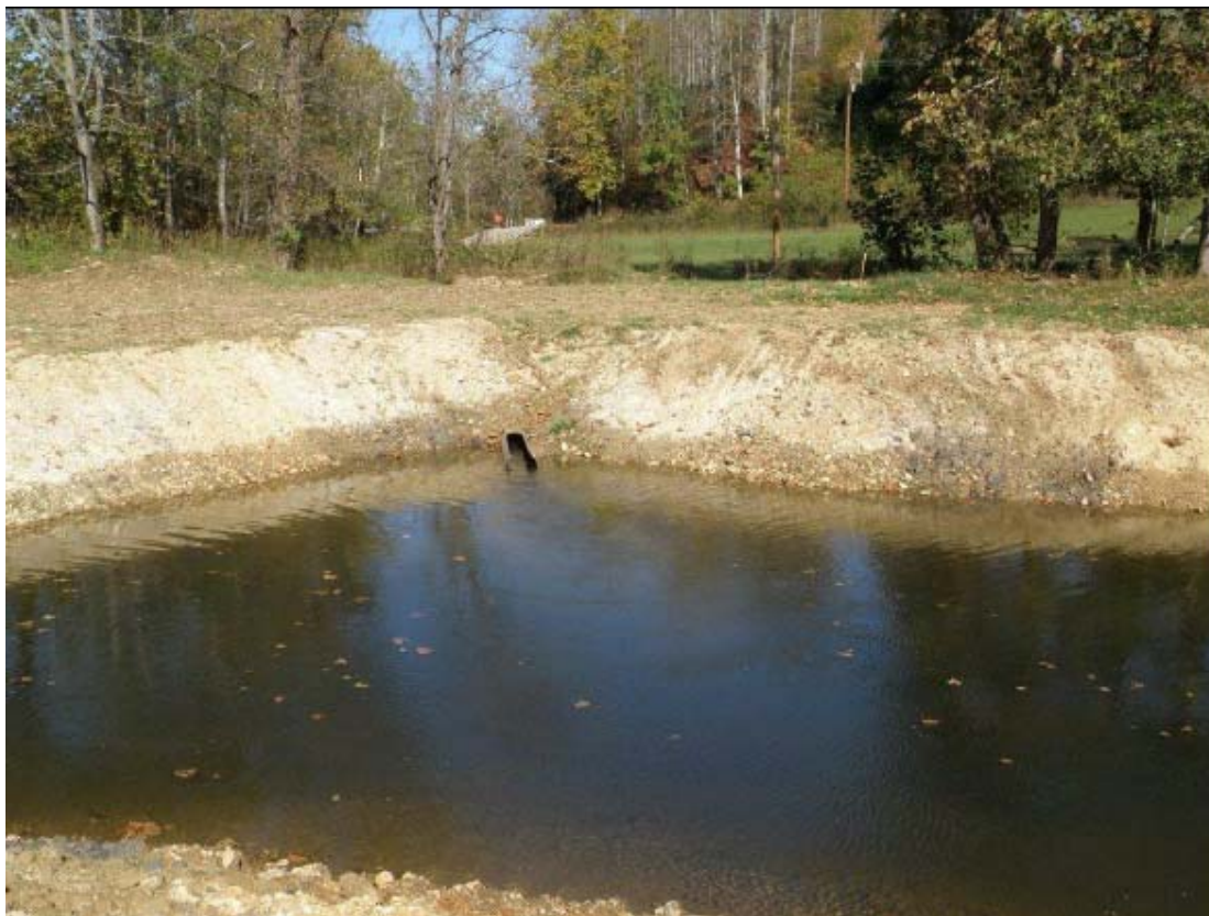
Photo 4.4 – Sediment basin located down-gradient of the slotted vortex pipe
