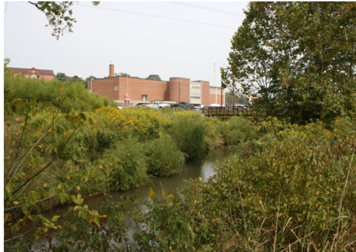
(c) Three years after restoration
