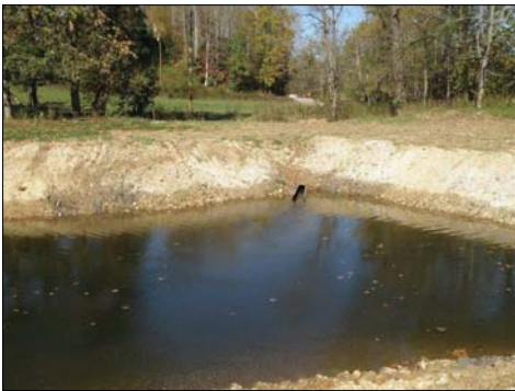
SEDIMENT VORTEX DISCHARGE INTO BASIN SCALE: NTS
