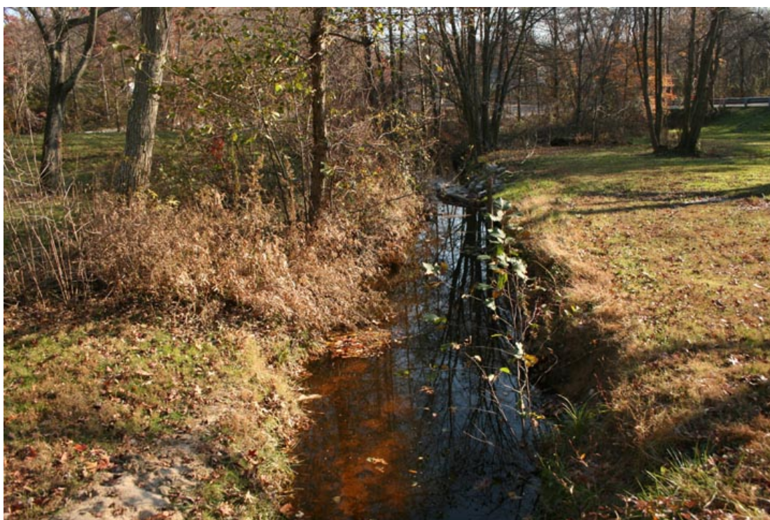
Photo 3.70 – Straightened lower section in park upstream of Trimble Road
