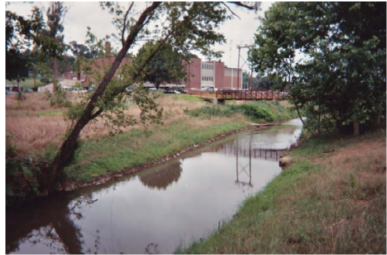
(b) Four months after restoration with toe benches. Note channel has been narrowed significantly.
