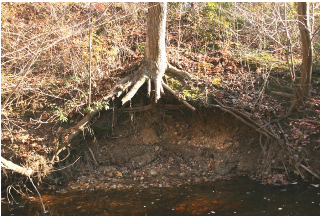
Photo 3.80 – Bank erosion along middle section
