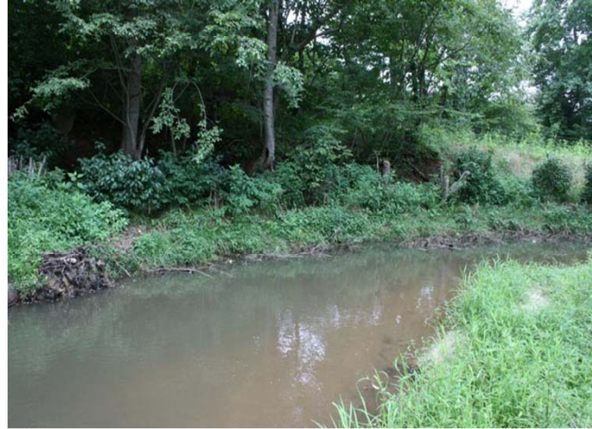
(b) Same reach one year after restoration. Note channel narrowed and bank reconstructed with toe wood to provide lateral control
