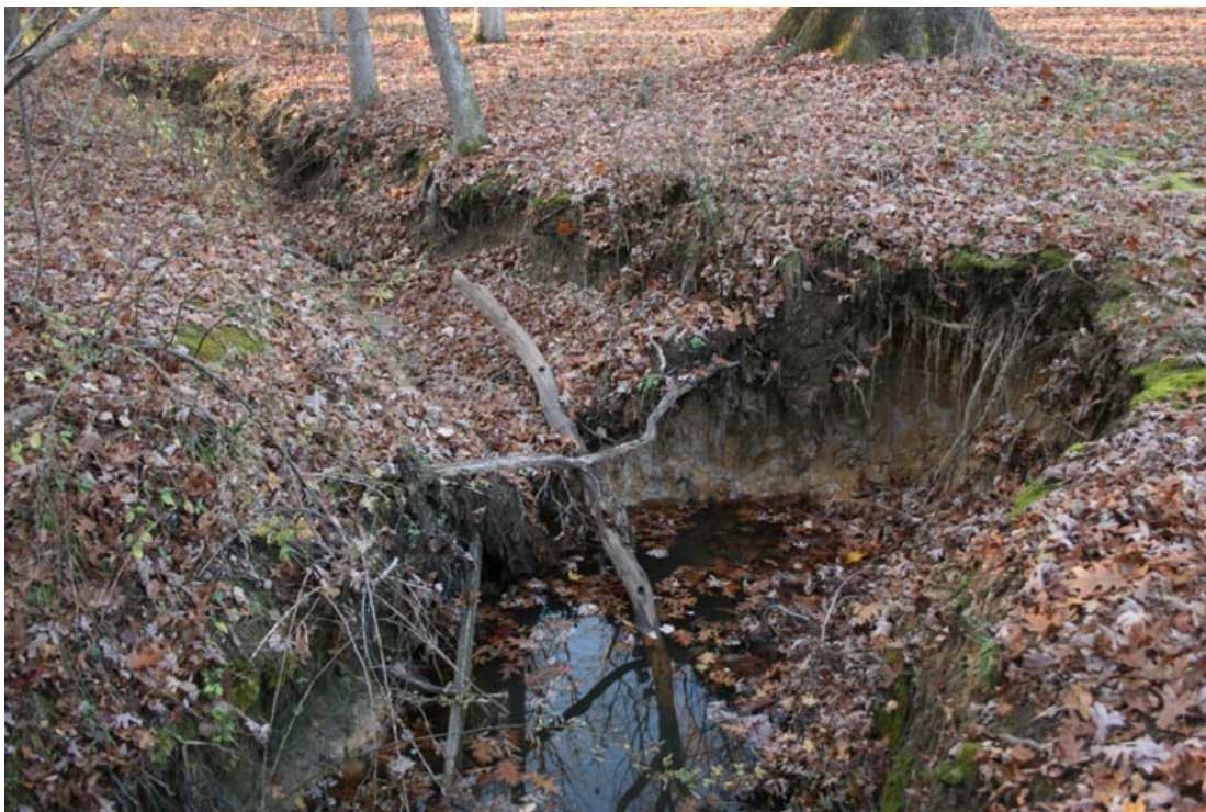
Photo 3.42 – Gully erosion and a 4 foot head cut along upper section
