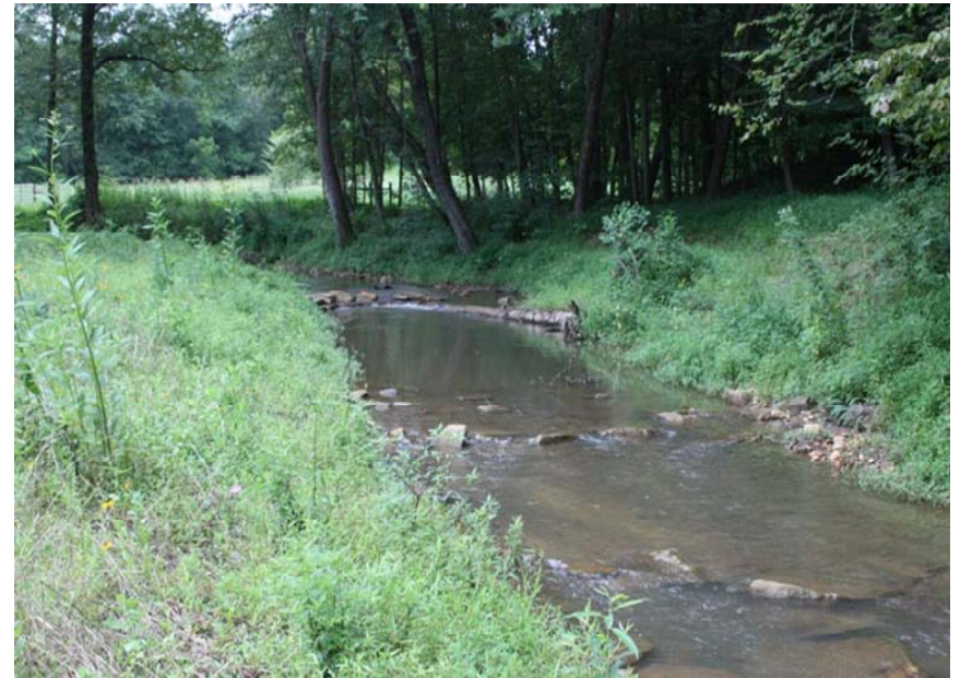
(b) Same reach one year after restoration. Note channel narrowed and constructed riffle and log-boulder J-Hook installed to provide vertical and lateral control
