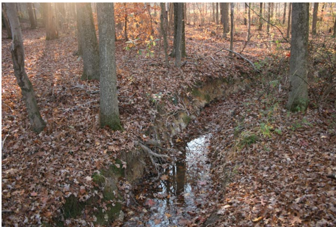
Photo 3.41 – Bank erosion along upper section
