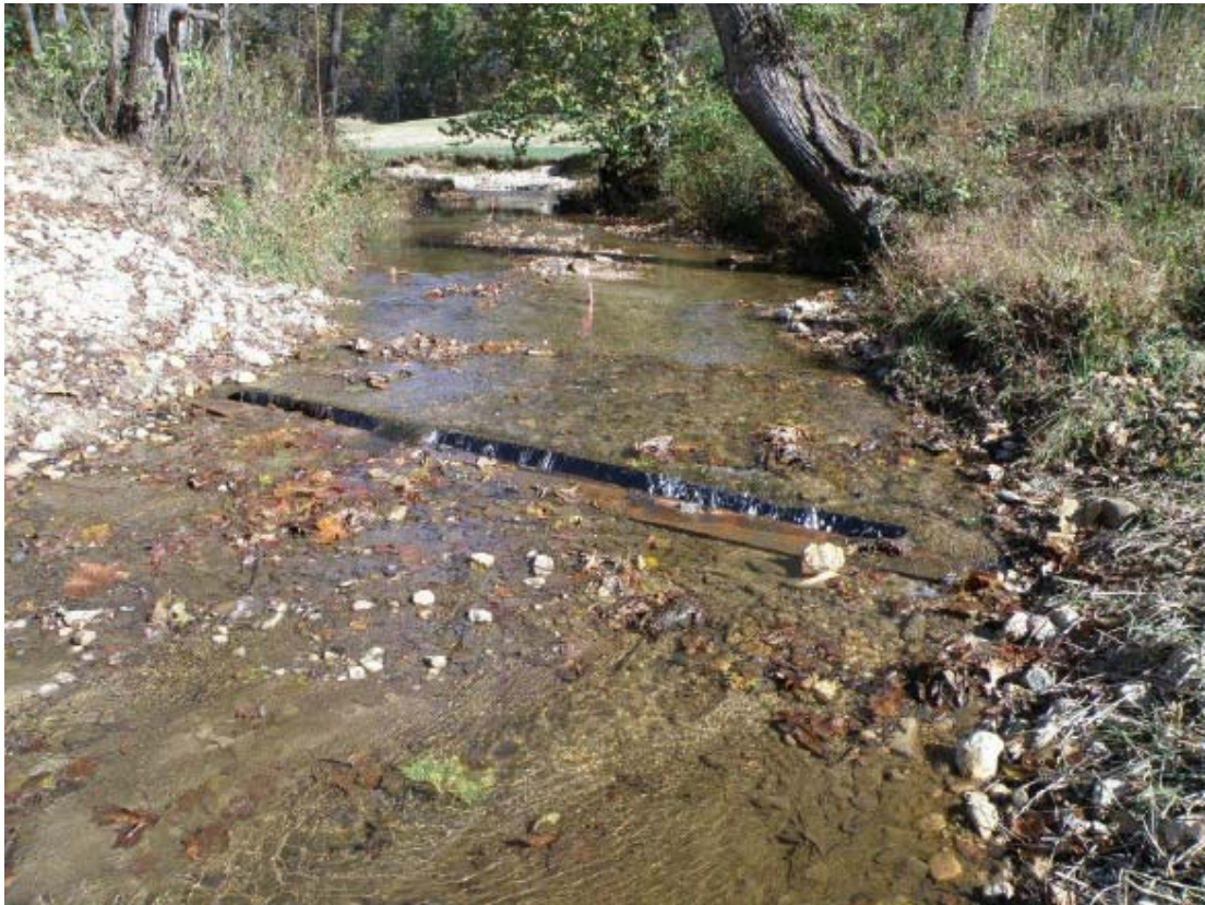
Photo 4.3 – Slotted vortex pipe
