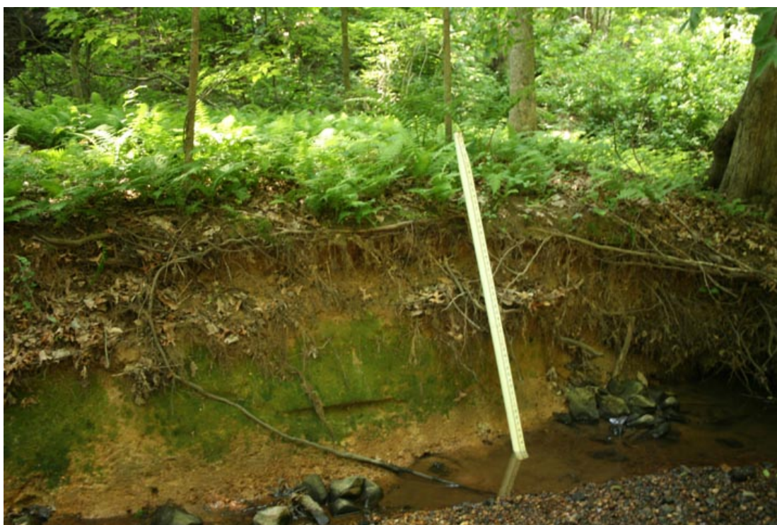
Photo 3.5 – Bank erosion along lower section
