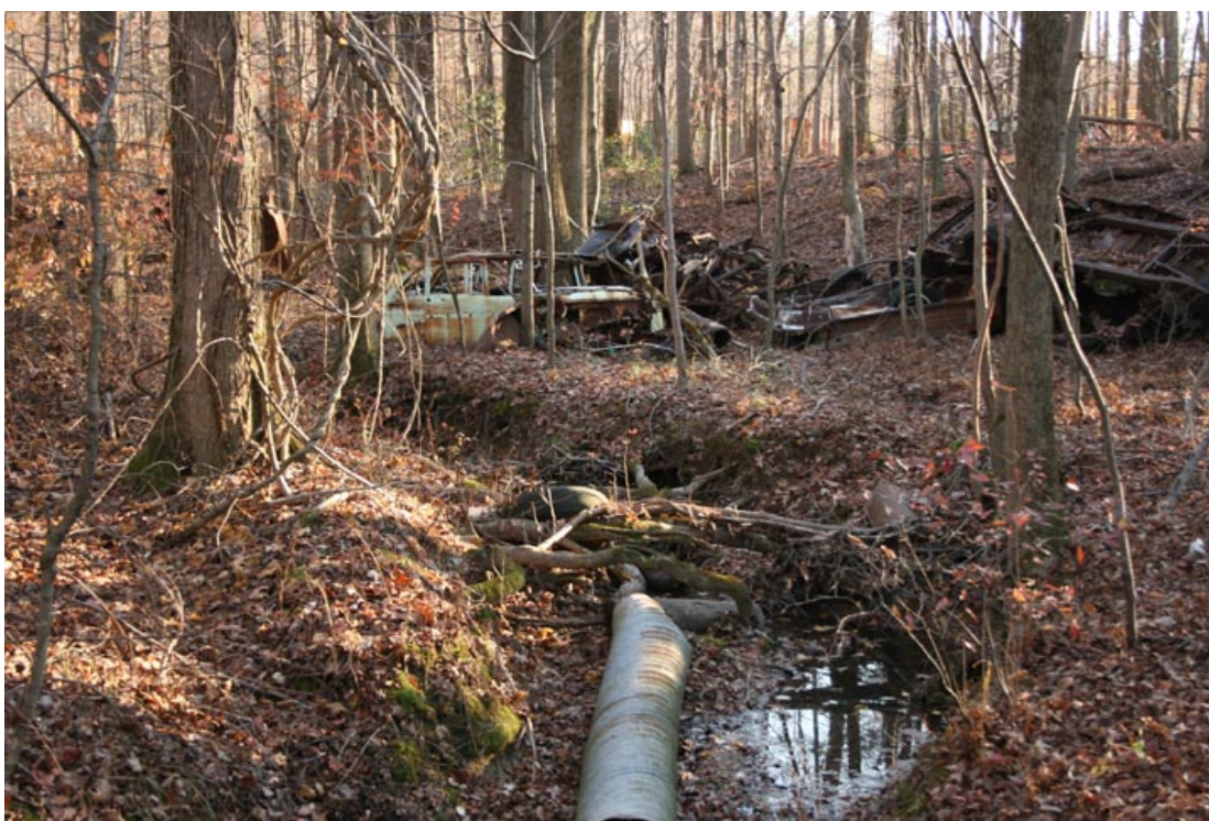
Photo 3.60 – Debris in channel and junk cars in floodplain lower section of South Tributary
