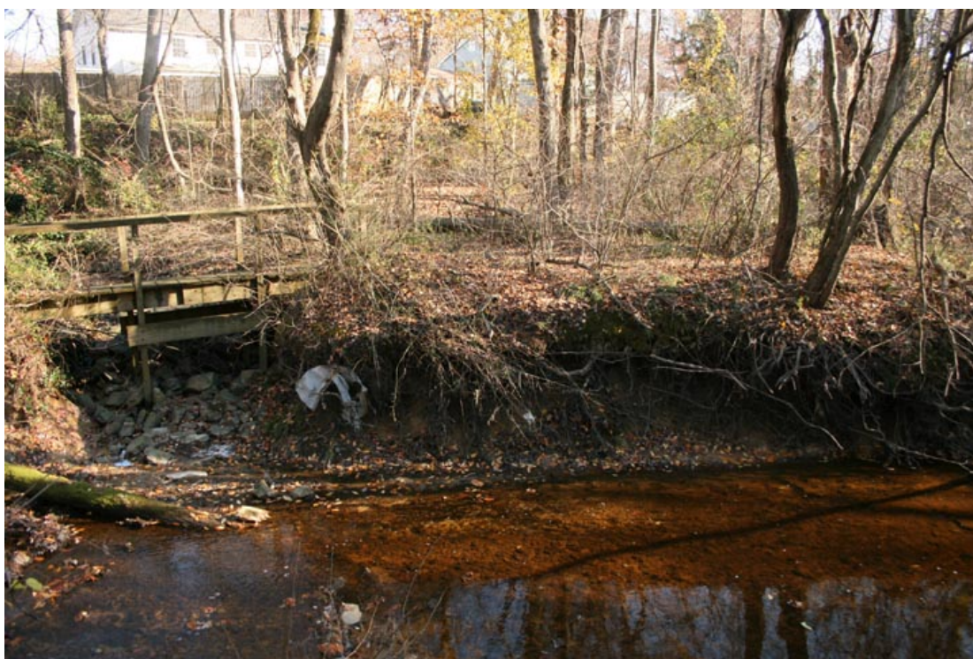
Photo 3.75 – Bank erosion and failing footbridge along upper section
