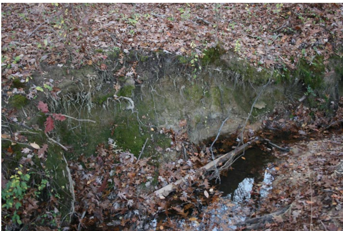
Photo 3.43 – Bank erosion along middle section
