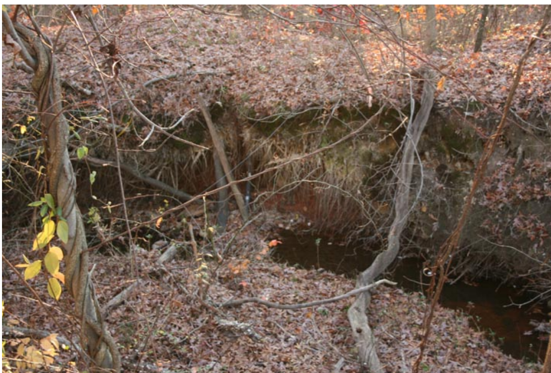
Photo 3.28 – Unstable G4 channel downstream of Route 40
