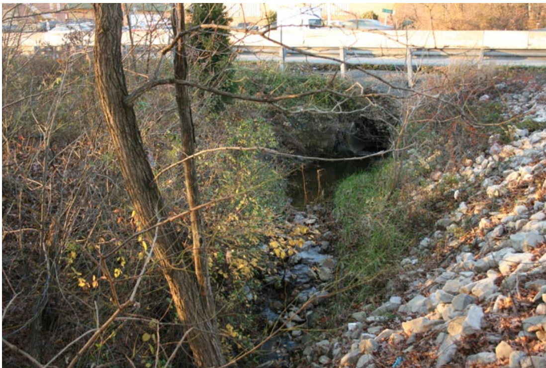
Photo 3.27 – Armored channel downstream of Route 40
