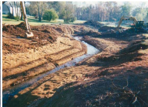
(b) Same reach during installation of soil fabric lifts
