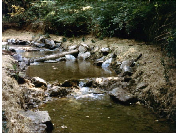
(b) Same reach immediately after stabilization with log/boulder step-pools and toe benches. Note bank trees not disturbed during construction
