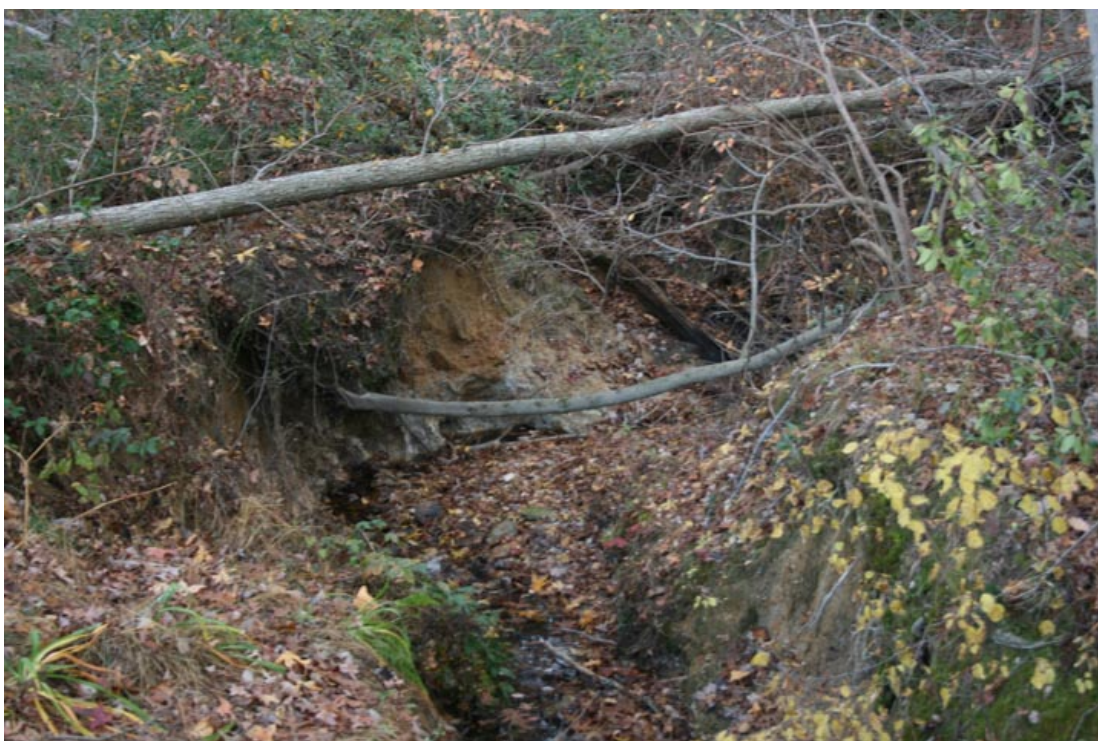
Photo 3.45 – Bank erosion along lower section
