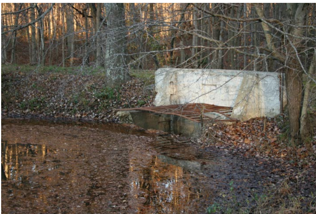
Photo 3.34 – Outlet structure of pond
