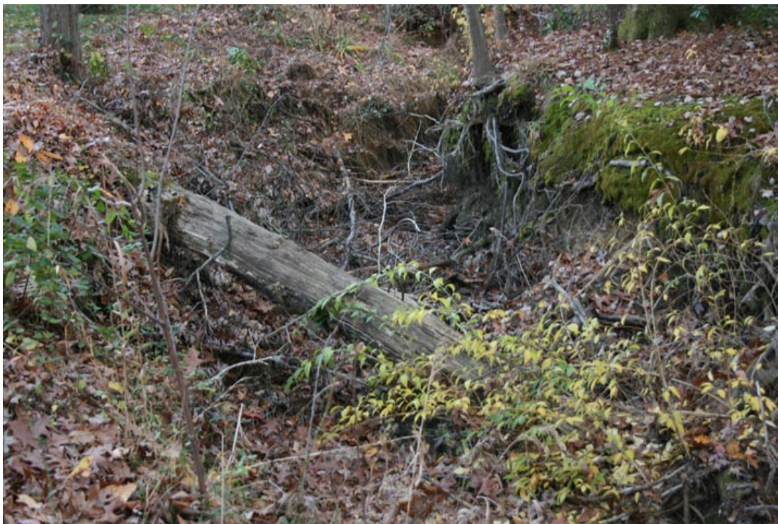
Photo 3.44 – Gully erosion and debris jam along middle section
