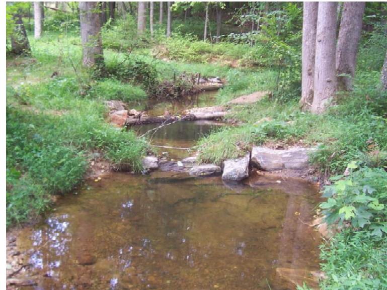
(b) Same reaches six months after restoration with log/boulder step-pools
