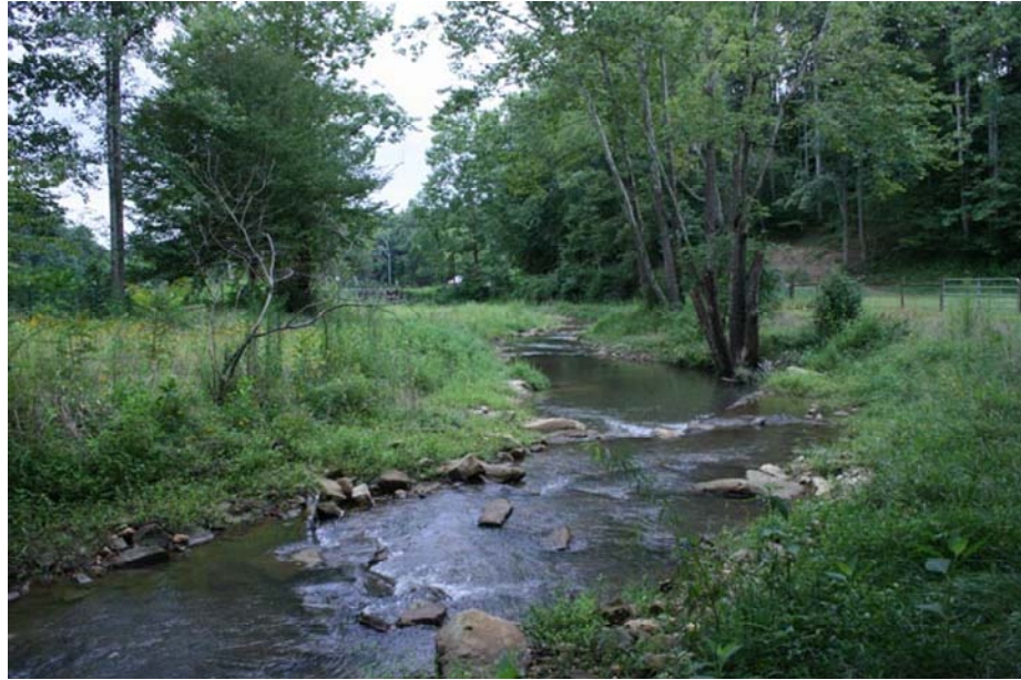
(b) Same reach one year after restoration. Note meander bends smoothed, channel narrowed and constructed riffle and log-boulder J-Hook installed to provide vertical and lateral control.
