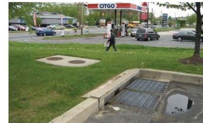
Existing inlet at east corner of lot
