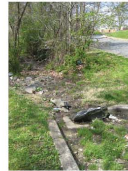
Riprap channel at southwest corner of parking lot
