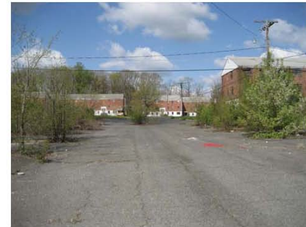
Existing pavement on Hawthorne Drive
