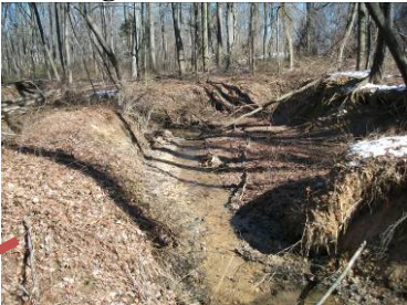
Existing: Over-widened Channel
