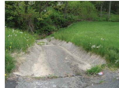
One of two existing channels from road into Sam's Branch
