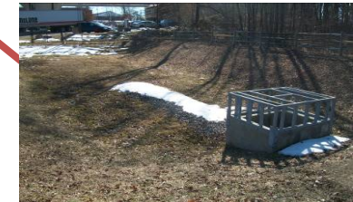
Existing Stormwater Pond at 7Eleven
