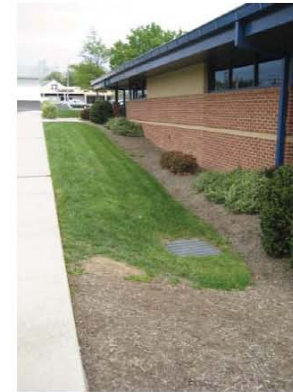
Existing swale and downspouts
