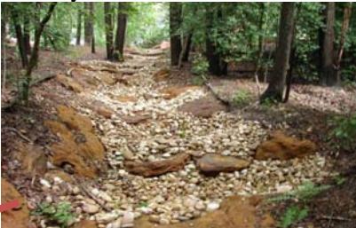
Proposed Regenerative Stormwater Conveyance
