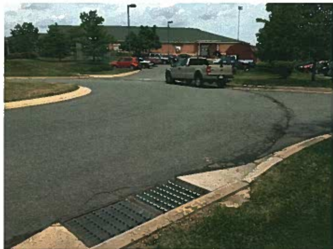
Existing inlet that captures stormwater runoff
