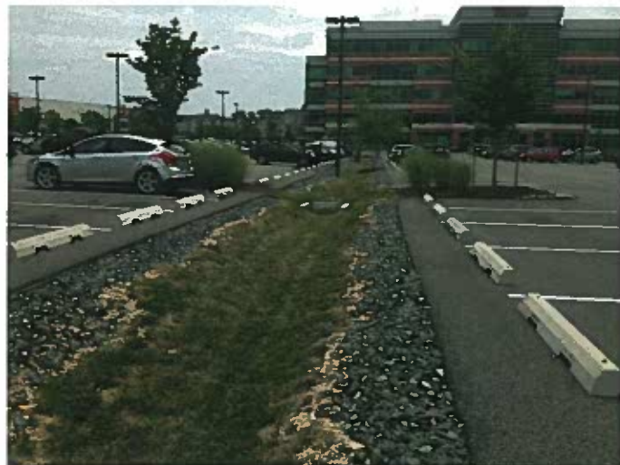
Existing swale with filter strips
