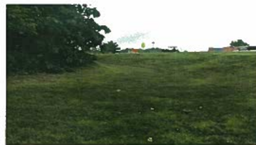
Grass channel that conveys runoff to the outfall
