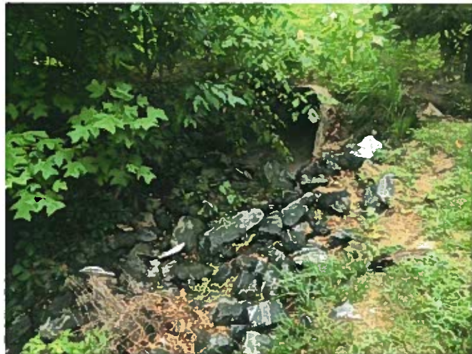
Existing outfall with riprap area
