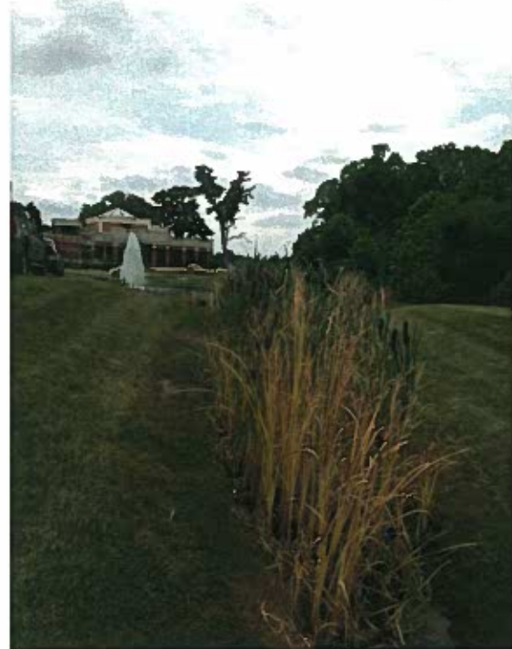
Existing Swale that conveys treated runoff to the pond
