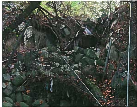
The existing wet pond outfall failure that contributes to the deterioration of Declaration Run Reach 2 collects stormwater from Baneberry Drive and Liriope Court.
