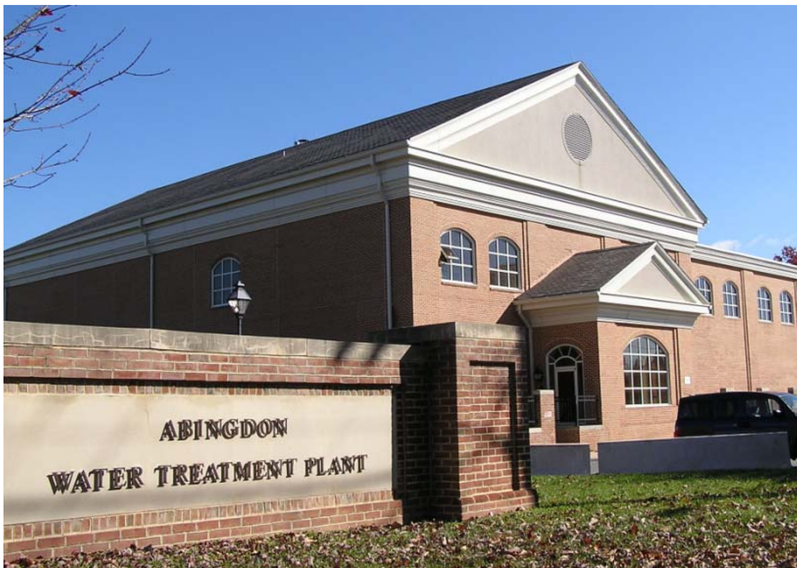
Abingdon Water Treatment Plant
