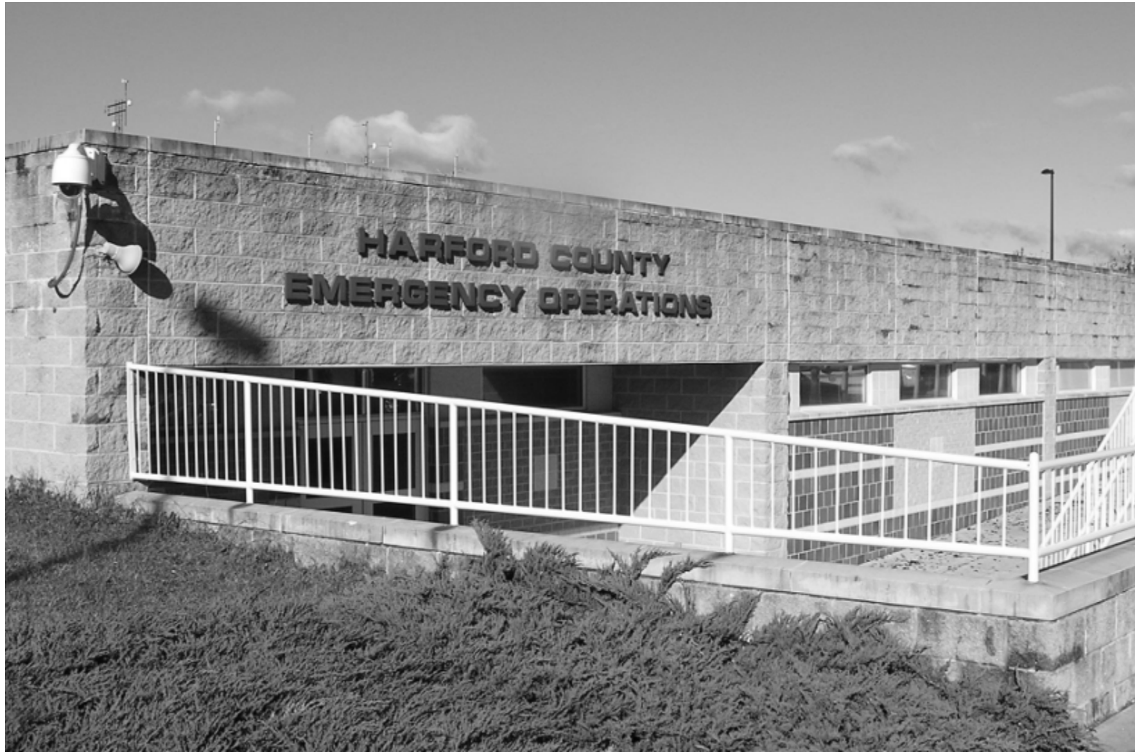
Harford County Emergency Operations Center
