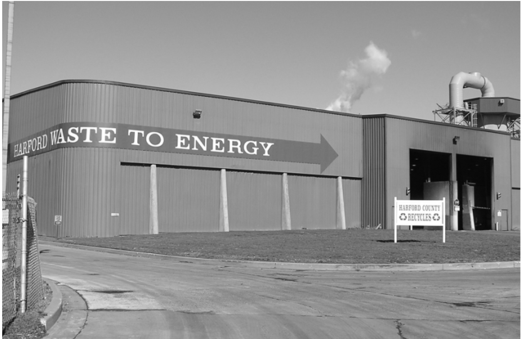
Waste to Energy Plant
