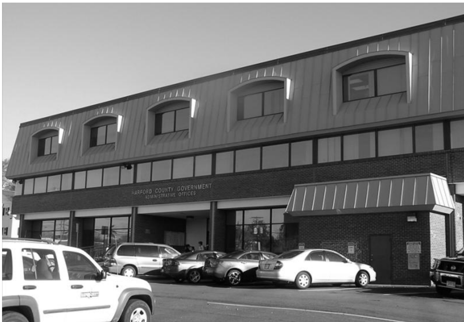
Harford County Administration Building
