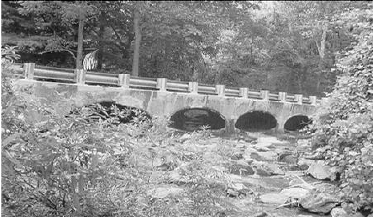
Ruffs Mill Road Bridge
