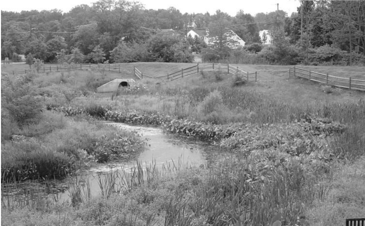
Mt. Royal Stormwater Management Facility
