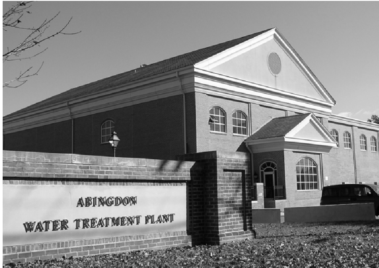
Abingdon Water Treatment Plant
