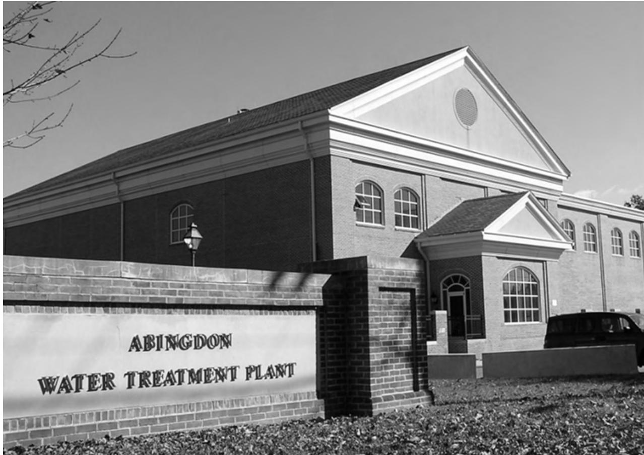
Abingdon Water Treatment Plant
