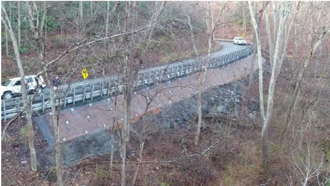
Section of Madonna Road slope stabilization project
