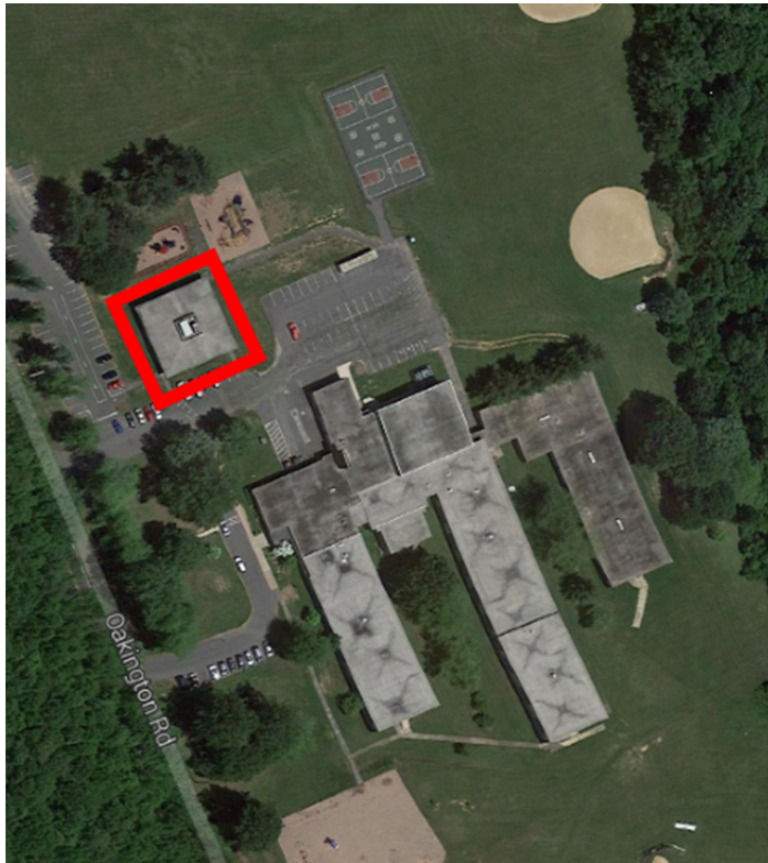
Figure 35: Roye-Williams elementary school with permanent out-building outlined in red
