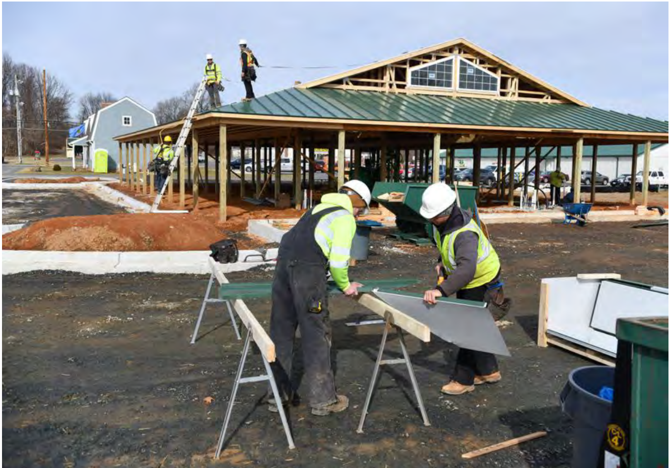
Workers install sections of a metal roof on the new Harford County agri-business incubator building, called The Grove, Thursday morning. The building is located next to the Harford County Agricultural Center in Street. (Matt Button / The Aegis/Baltimore Sun Media)
