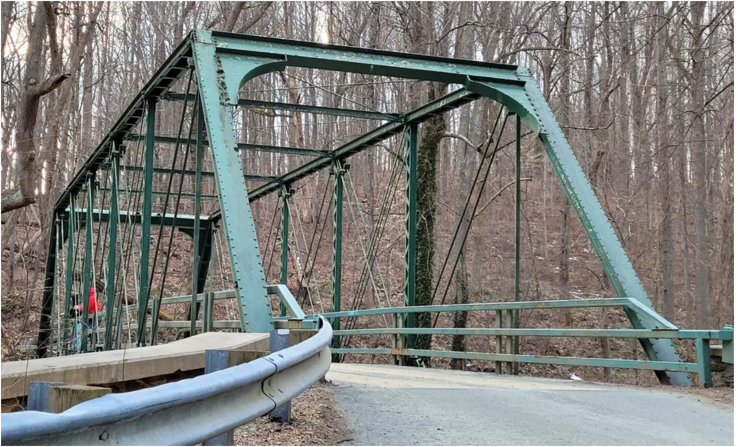
Bottom Road Iron Bridge, 1886 (BA-961), Fallston is a wrought iron Pratt through truss.
