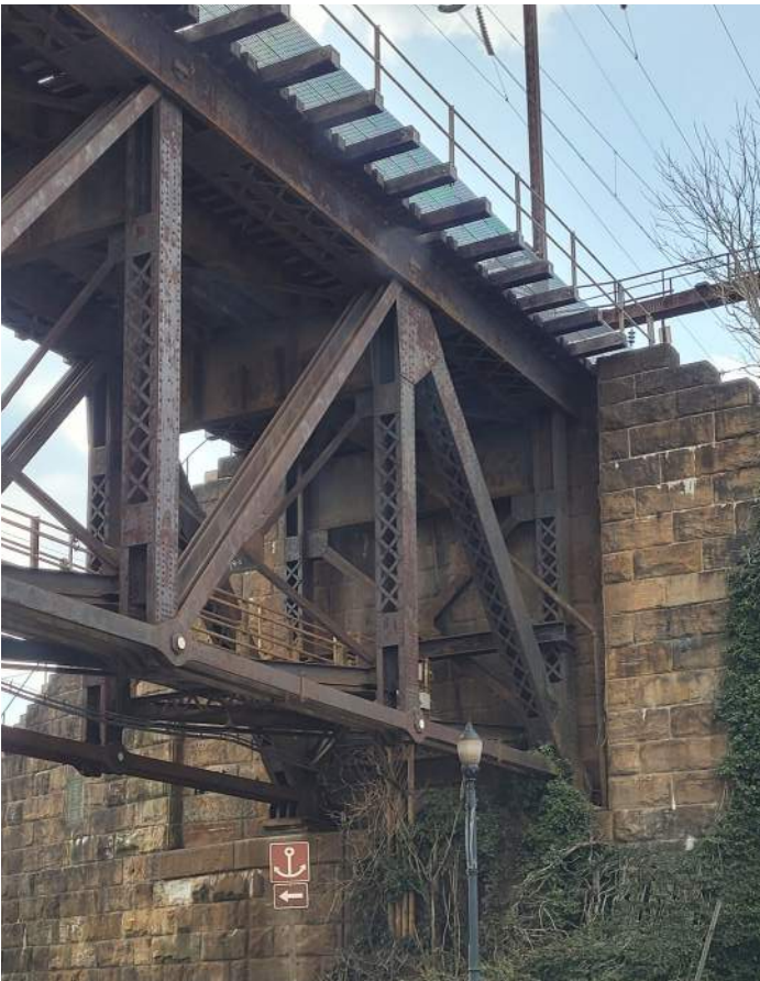
Amtrak Railroad Bridge over the Susquehanna River, 1906 (HA-1712), Havre de Grace is a deck-and-through truss bridge made of steel with stone piers.
