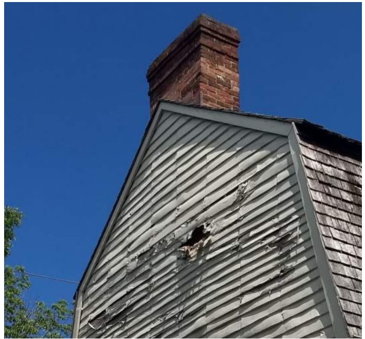
Adding insulation to the wall cavity can potentially cause harm to the historic fabric if moisture becomes trapped in the walls. HCG File Photo.
