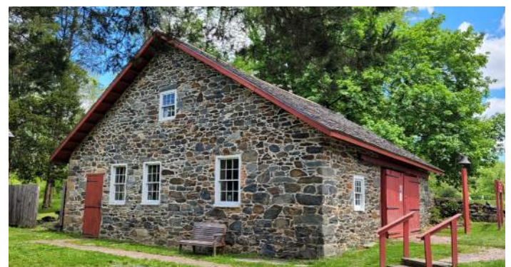
The rubble-fieldstone walls of the Jerusalem Mill Blacksmith's Shop (HA-435), Joppa are an important character-defining feature.
