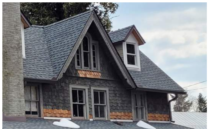
Wood shingle repairs to the Millstone Farm (HA-1693), Darlington.
