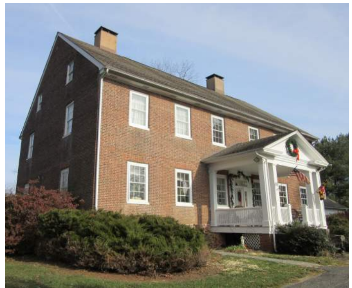
Sophia's Dairy, 1768 (HA-5), Belcamp is constructed of Flemish bond brick walls. HCG File Photo.
