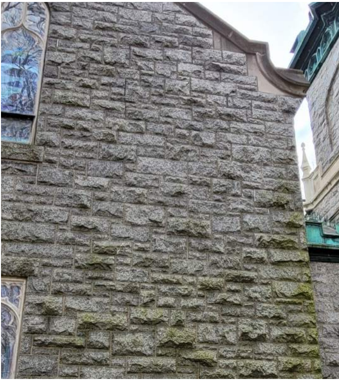
Havre de Grace United Methodist Church, 1902 (HA-1125), Havre de Grace has rock-faced ashlar walls made of Port Deposit granite.
