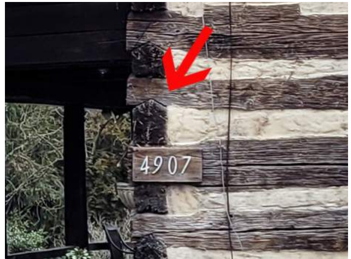
The Jolly Acres Old Mill in Norrisville is constructed using "V" notching.
