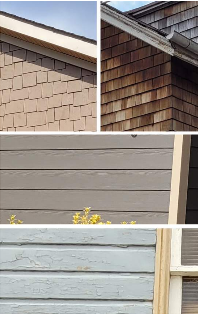
Modern synthetic materials (upper left and middle) do not typically have the same texture and thickness as traditional materials.
