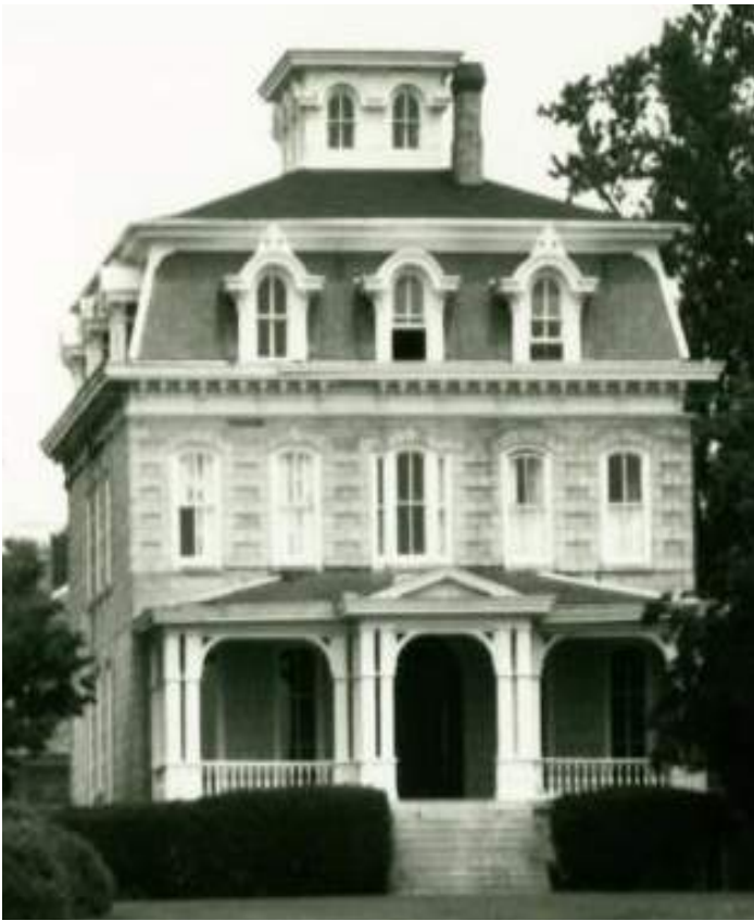
The mansard roof of Fair Meadows, 1868 (HA-1067), Creswell (no longer extant) includes dormers with rounded tops and a cupola at the top. HCG File Photo.
