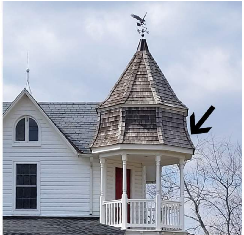
Edward L. Wilkinson Farm, late 19th century (HA-1569), Level (left image courtesy of Maryland Historical Trust). The roofing on the lower portion of the tower has been replaced with wood shingles matching the upper portion.
