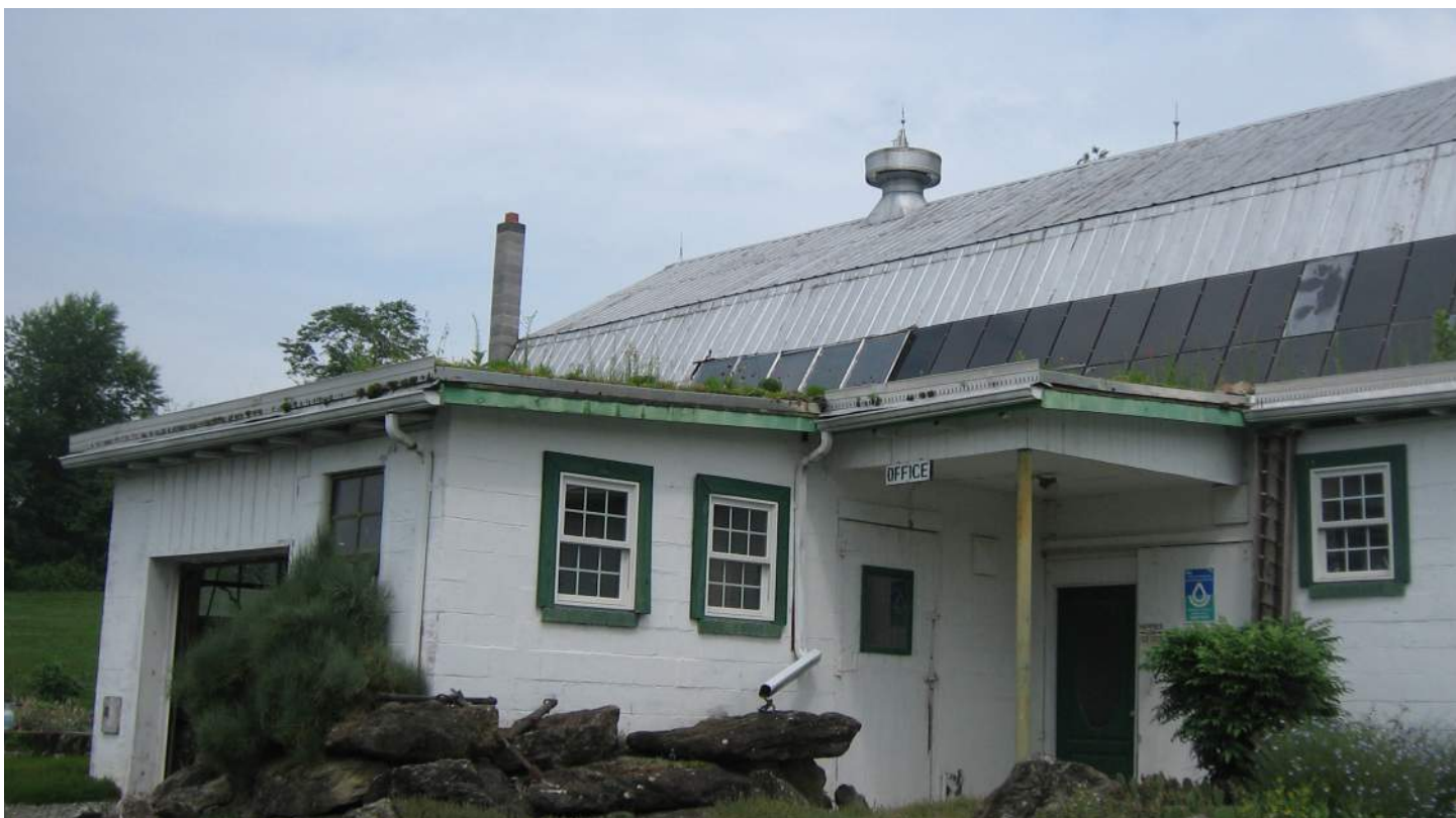
Natural vegetation is used on this flat area of green roof at the mid-twentieth century dairy barn at Emory Knoll Farm. Photovoltaic panels are also used at the lower edge of the gambrel roof. Image courtesy of Jen Wilson.
